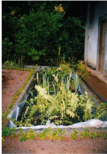
Figure 26: The vertical flow planted gravel filter unit of the Swiss Residence Hotel after commissioning
