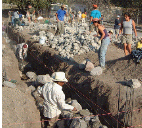
Figure 21: Building zapatas
