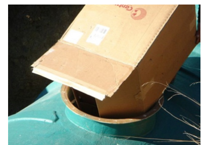
PHOTO 6 BIOMEDIA POURED INTO THE TWO AEROBIC CHAMBERS
