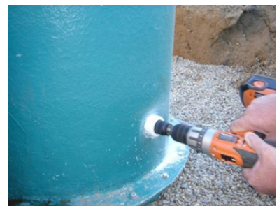
PHOTO 10 CUTTING HOLE FOR BULKHEAD FITTING
