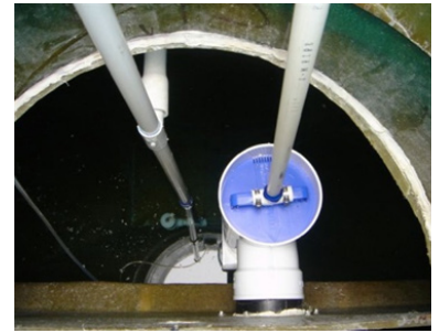
PHOTO 51 ATTACH HANDLE TO EFFLUENT FILTER
