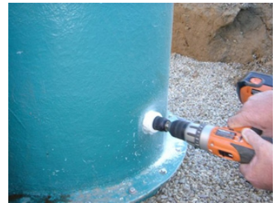
PHOTO 36 CUTTING HOLE FOR DISCHARGE ASSEMBLY
